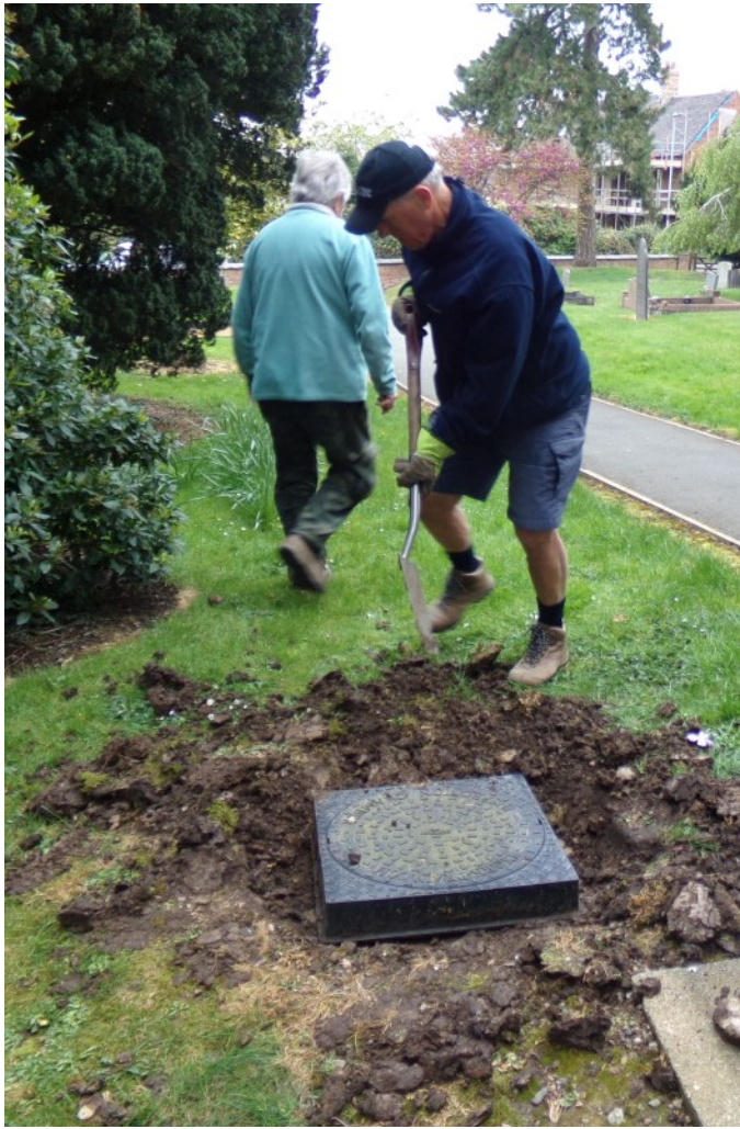
Levelling inspection chambers
